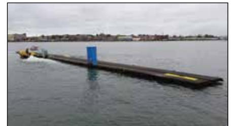
The steel and concrete breakwater built by Boston Bridge and Steel arrived at the marina via water, pushed by work boats across the harbor.
